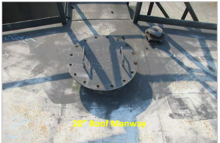
Stairway landing, 20" Roof Manway, 8" Gauge Port
